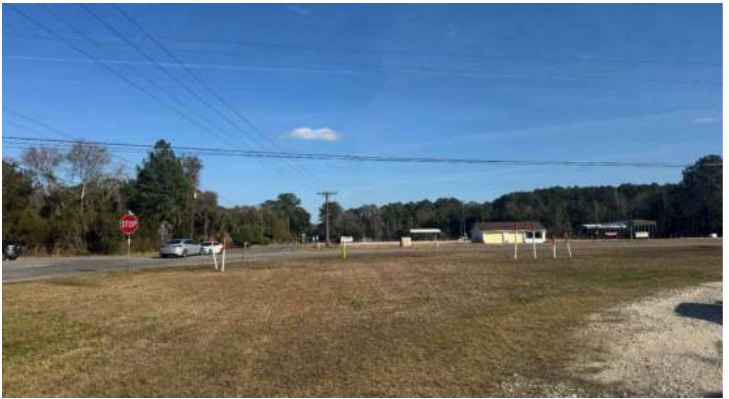
PHOTO # 17 View of southeastern adjoining US Highway 17 and Colerain Road intersection. View facing east.
