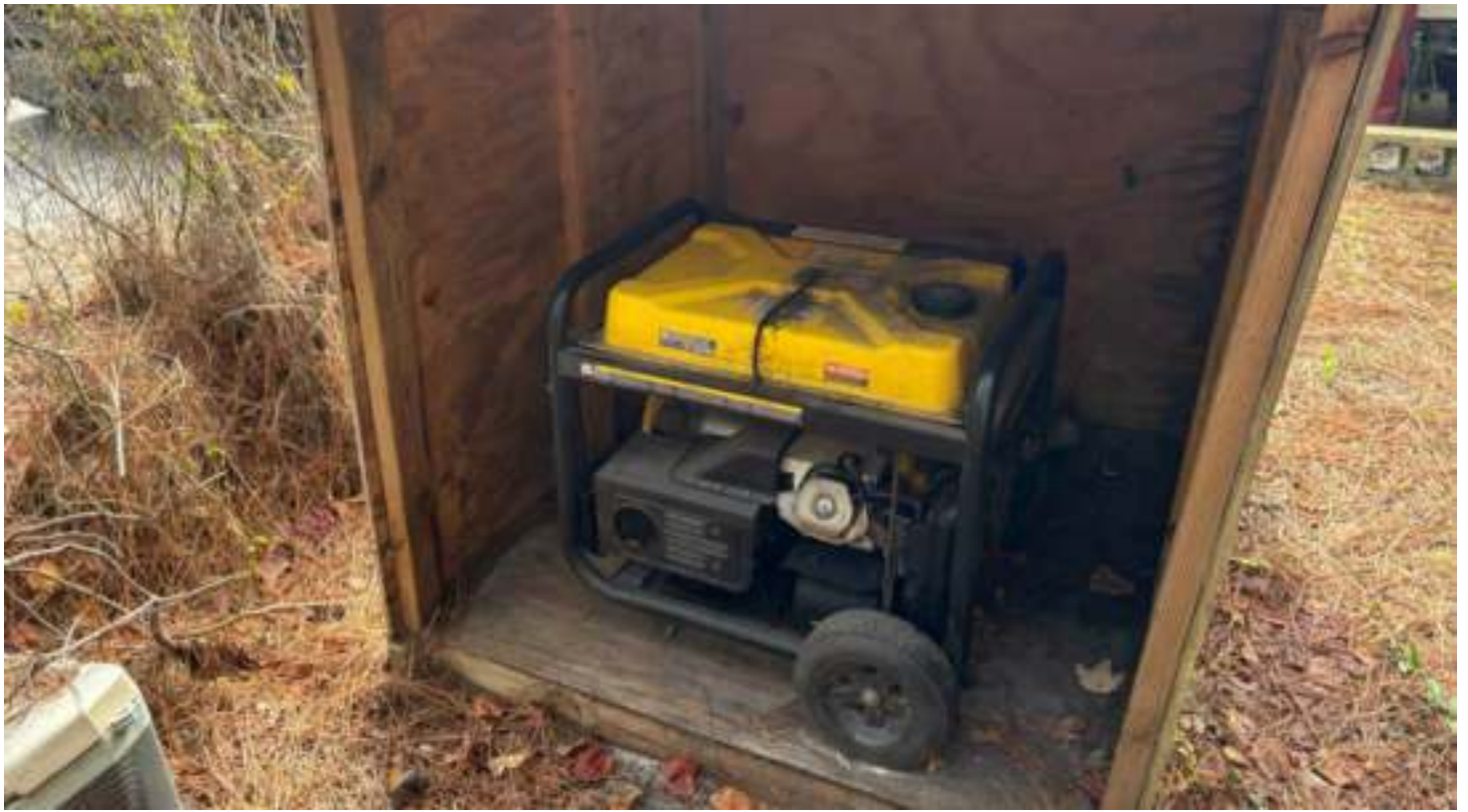
PHOTO # 33: View of a generator in the hunting camp on the northern interior portion of the subject site. View facing south.
