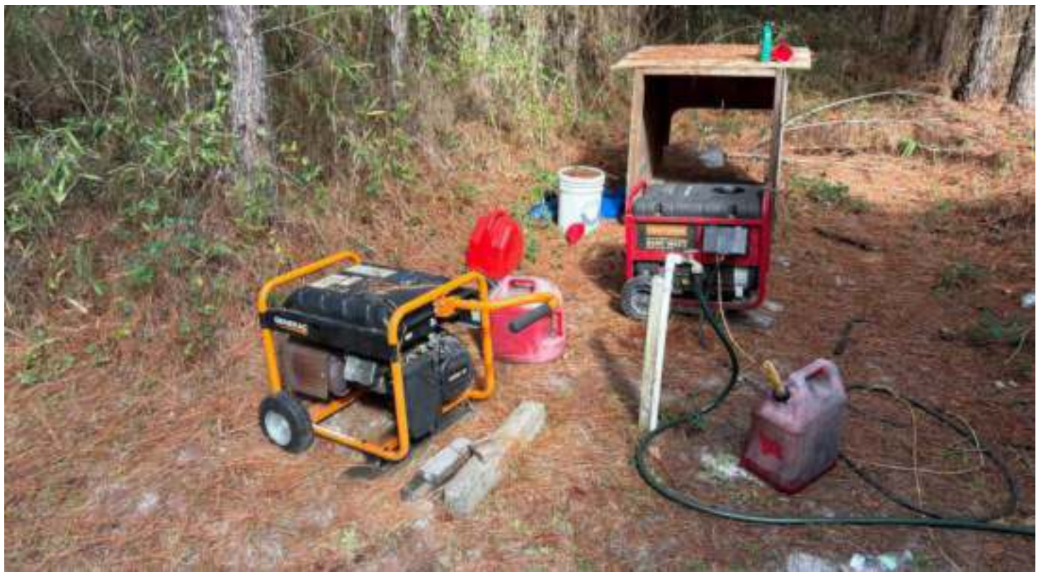
PHOTO # 24: View of two generators and gasoline containers in the hunting camp on the northern interior portion of the subject site. View facing north.
