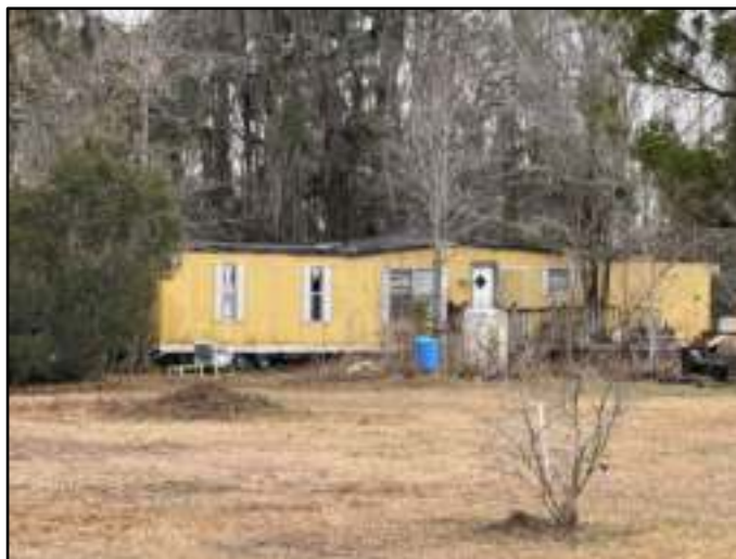
Figure 5-43. 0 US Highway 17, facing southwest.
