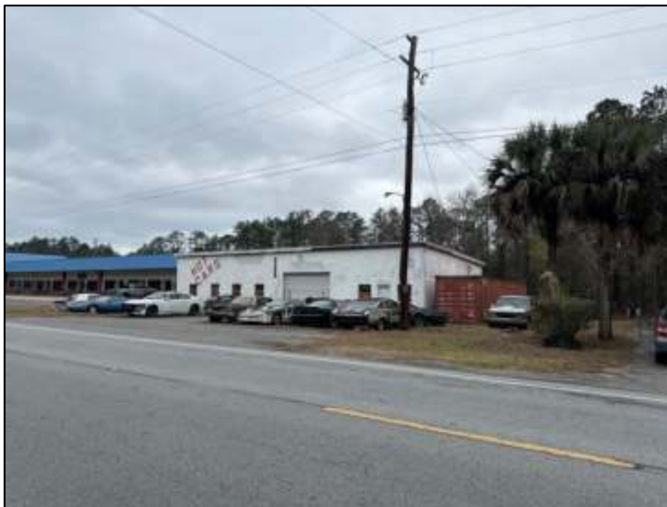
Figure 5-39. 5711 US Highway 17, facing southwest.
