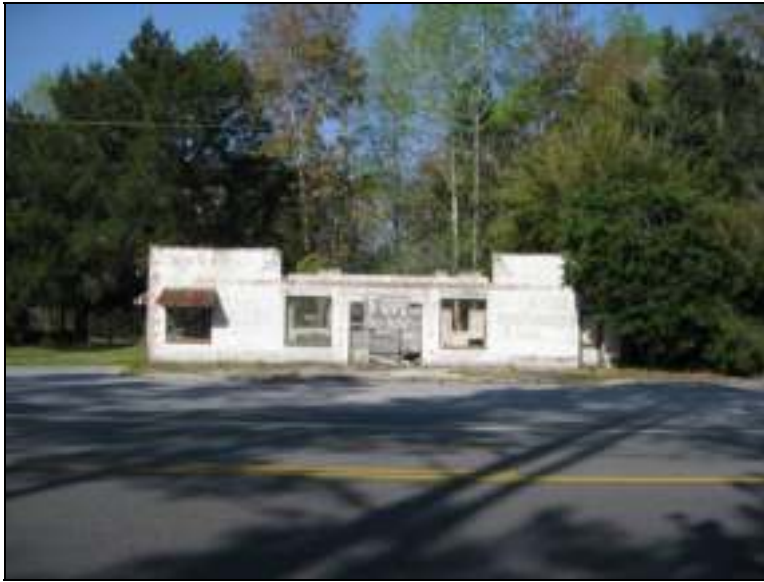
Figure 10: Structure 6, Facing West
