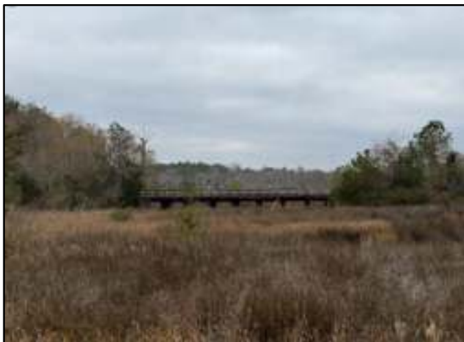
Figure 5-36. Railroad Bridge 596.5, facing southwest.
