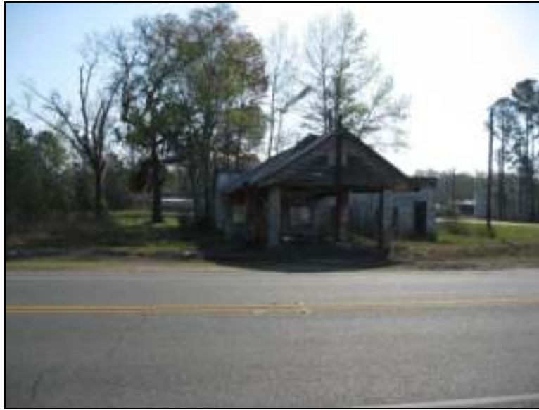
Figure 16: Structure 9, Facing West
