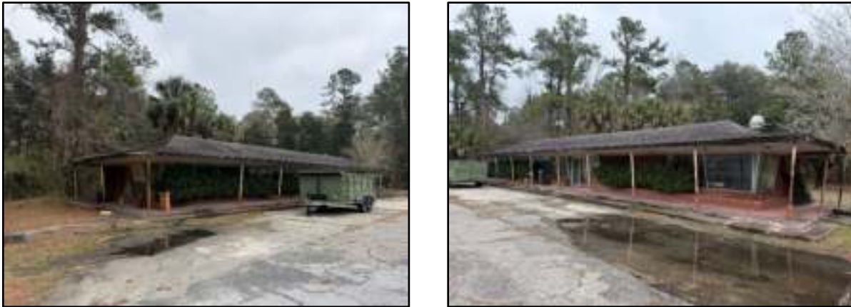
Figure 5-30. View of the historic-age building located at 5990 US Highway 17, view facing northeast.
