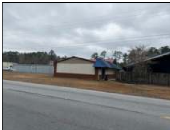
Figure 5-38. 5685 US Highway 17 facing southwest.
