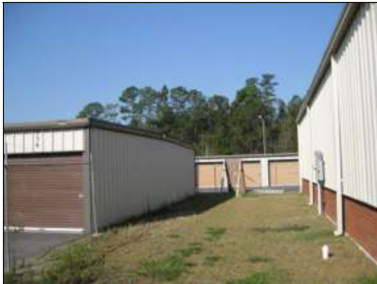
Figure 23: From Structure 12, Towards Subject Parcel, Facing West
