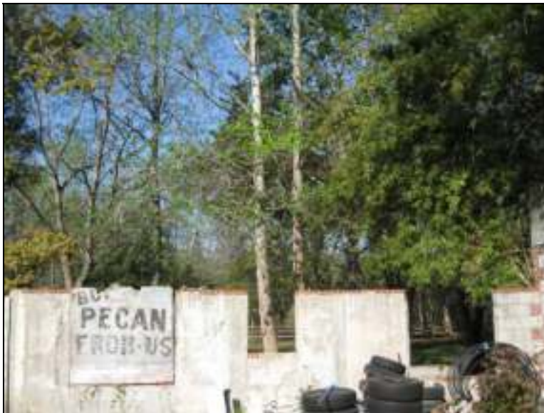
Figure 11: From Structure 6, Towards Subject Parcel, Facing West
