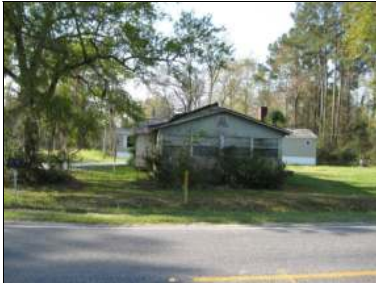
Figure 24: Structure 13, Facing South
