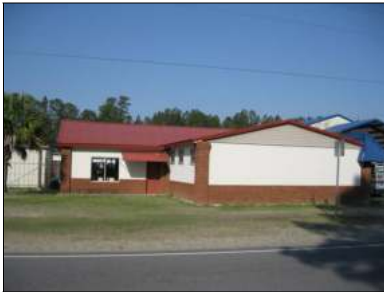
Figure 22: Structure 12, Facing West
