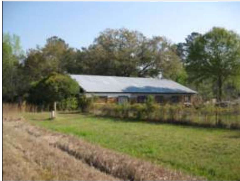
Figure 14: Structure 8, Facing Northeast
