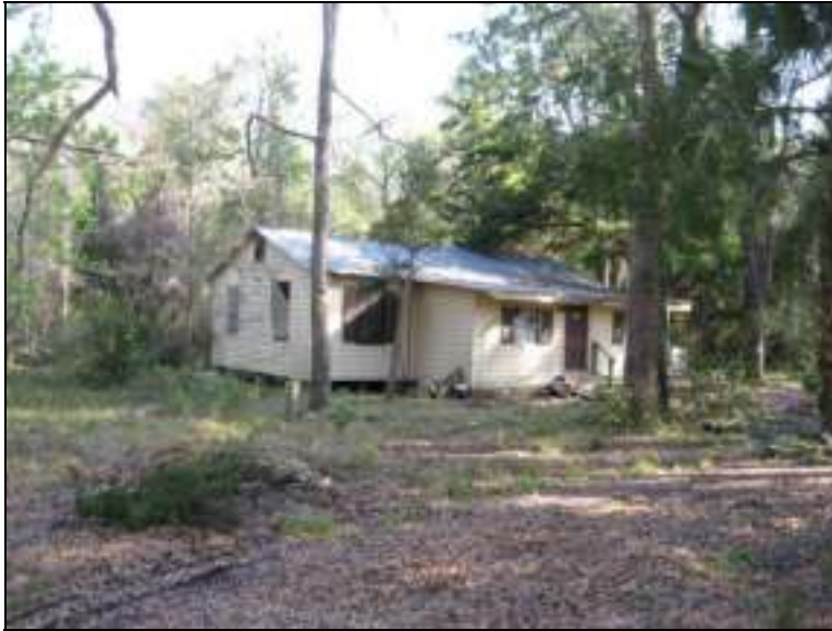
Figure 20: Structure 11, Facing North
