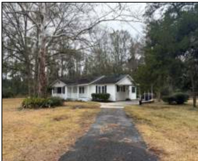
Figure 5-44. 8005 US Highway 17, facing southwest.
