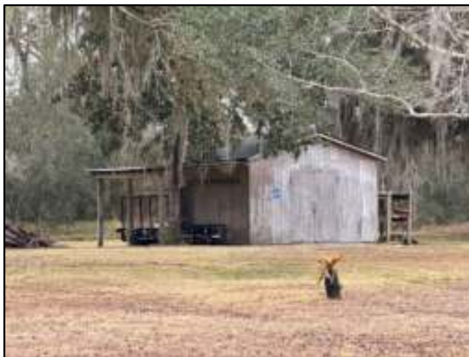
Figure 5-42. 7405 US Highway 17, facing southwest.
