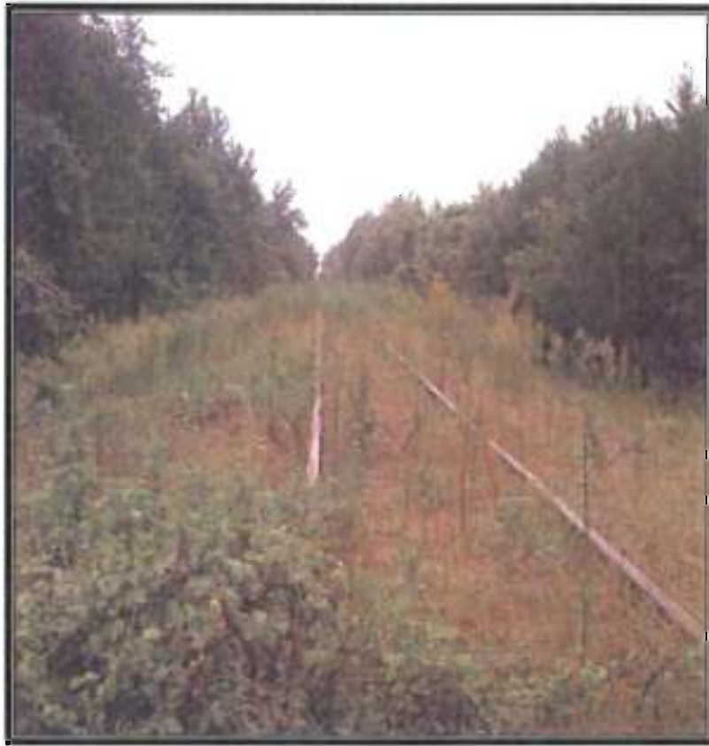
Figure 6.33: South View of the Abandoned CSX Railway
