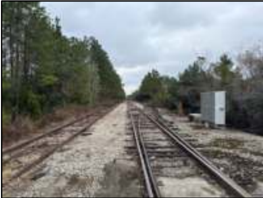
Figure 5-32. View facing north at Colerain Road.
