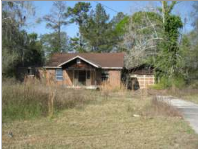
Figure 4: Structure 2, Facing West
