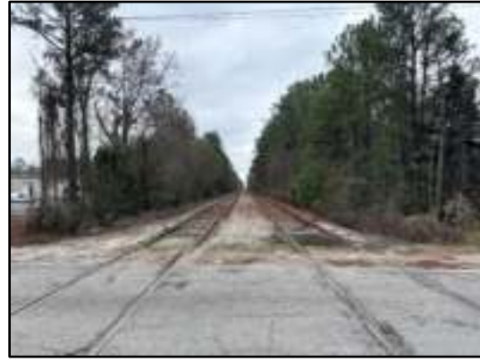
Figure 5-33. View facing south at Colerain Road.
