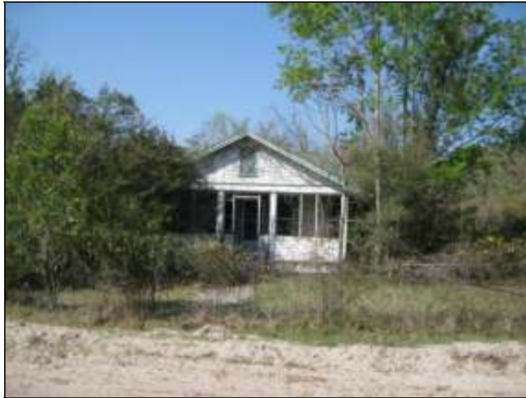
Figure 2: Structure 1, Facing West
