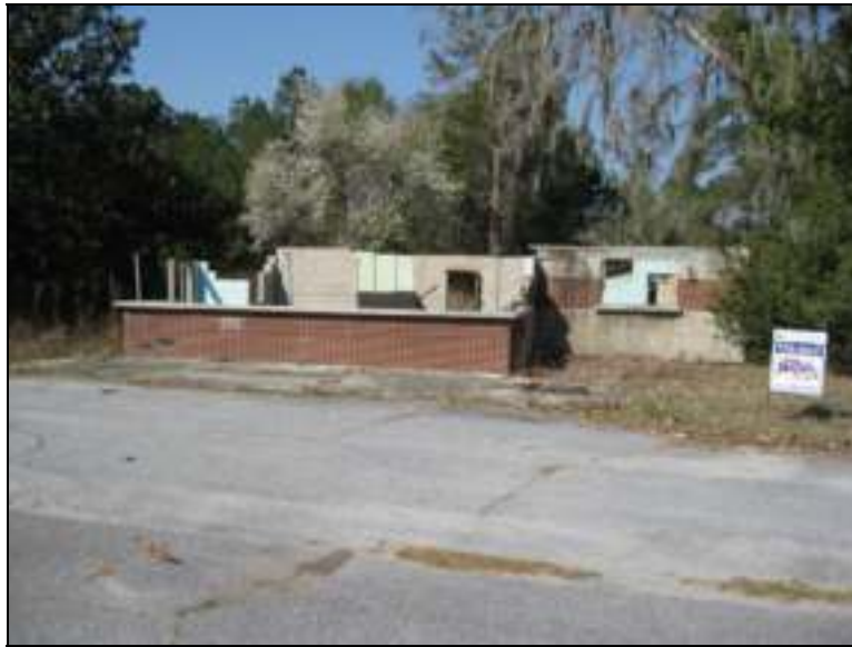
Figure 6: Structure 3, Facing West
